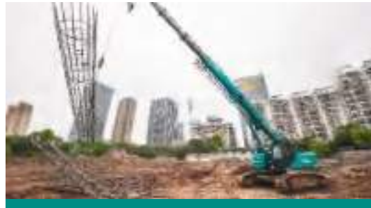
SWTC5 construction in the UK
