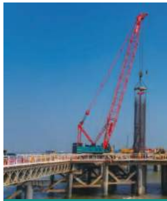
SWQY85 construction for Shenzhen-Zhongshan Bridge
