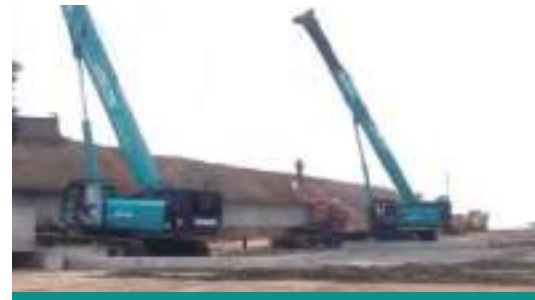
SWTC75 construction for Qijing bypass expressway in Yunnan Province
