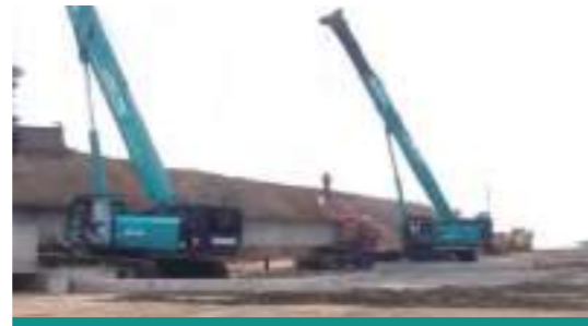
SWTC75 construction for Qujing bypass expressway in Yunnan Province
