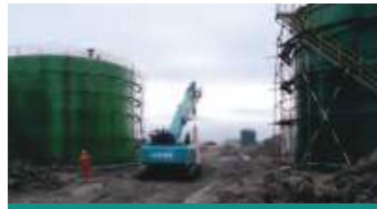
SWTC25 construction in Daqing oilfield site with traveling with load operation
