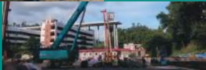
SWTC55B construction in Shenzhen Hongling High School
