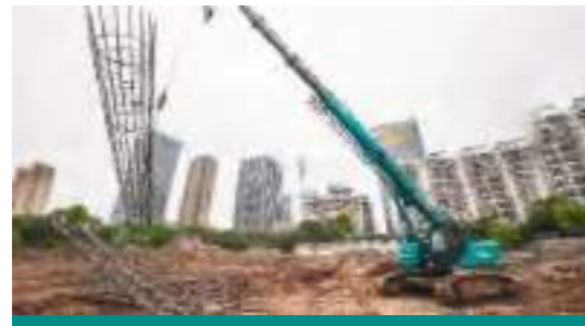
SWTC5 construction in the UK
